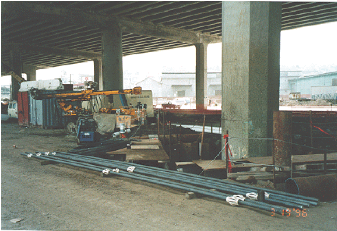
Figure 8-3. Storage of Reinforcing Steel.
