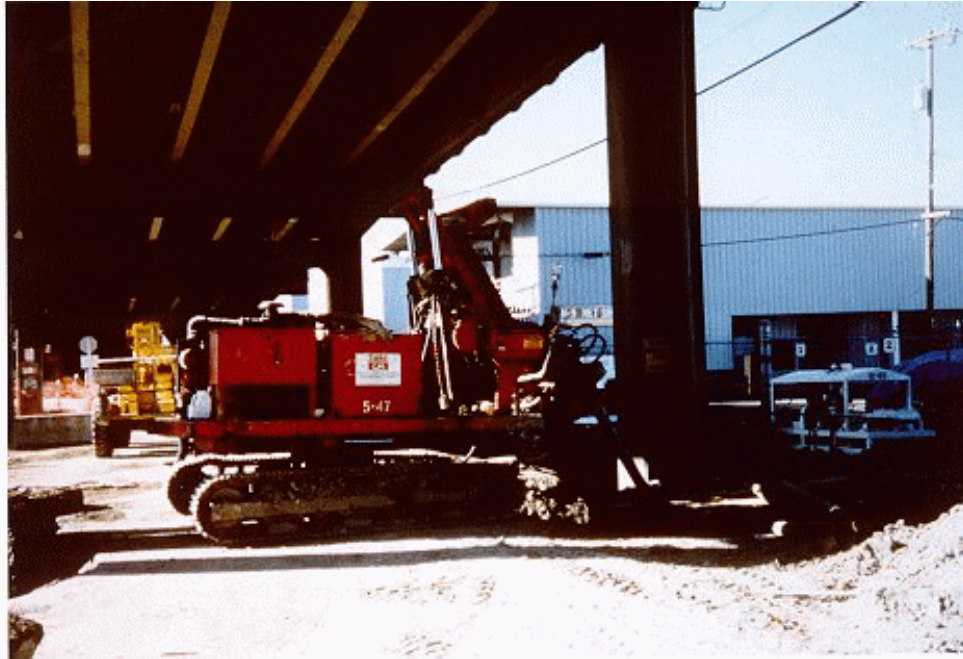
Figure 3-6. Underpinning of West Emerson Street Viaduct, Seattle, Washington.
