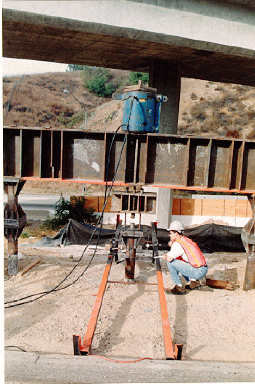
Figure 7-5. Tension Load Test Set-Up.
