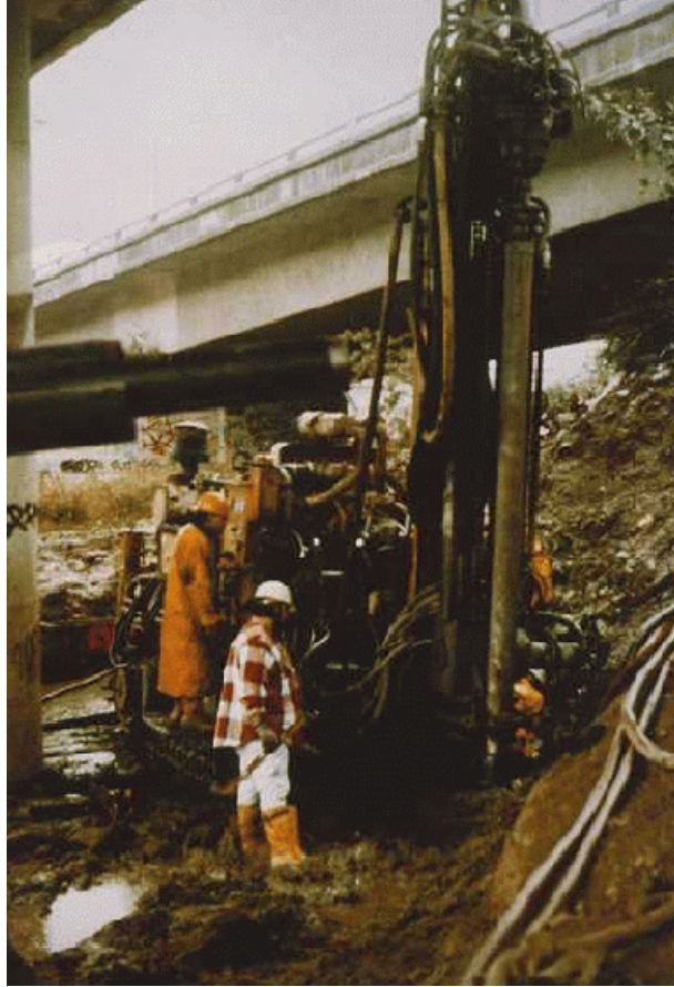
Figure 3-8. Seismic Retrofit of I-110, North Connector, Los Angeles, California.
