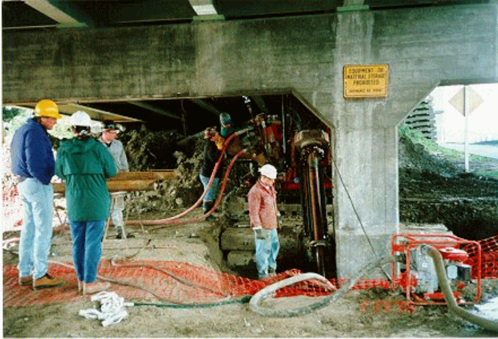
Figure 3-2. Low Headroom Micropile Installation.
